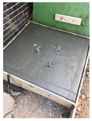
After the cement was poured it was time to strip some of the upper bracing off and skim the surface with a trowel to smooth it out and to put on a rounded edge to the block.
