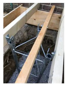
This is especially critical when having a pumper truck delivering concrete under pressure. It is possible to dislodge the base by the power of the pour. Each of the upright portions of the base were screwed into a 2x4 to hold the base in its position. The 2x4s were then nailed to the form walls.
