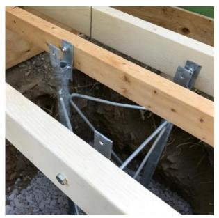
I ran two plumb bobs to make sure the cage would fit properly by the garage. I also made sure my angle of attack would allow the tower to be lowered through the open gate onto the backyard.
