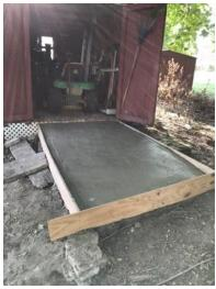
Cement needs time to cure. For the first week, I needed to cover the cement with a damp covering to help slow the drying of the top layer before the inside portion of the cement does. A daily dose of misting water was enough to do the trick. Boy that cement got warm too!
