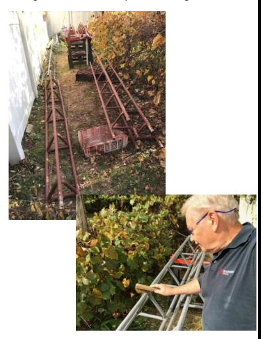
Next I moved on to refurbishing the tower sections I have. I needed to wire brush the old paint off as much as could be done. Then I painted them with a brown Rustoleum rust primer. Then with an exterior coat.
