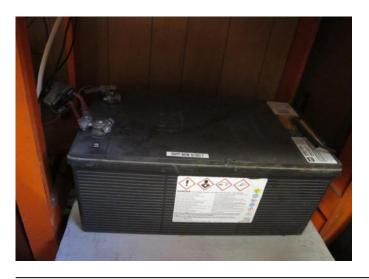
tery also helps minimize voltage sag along the bus. It is connected via a fuse. (You can also see part of a dummy load in the picture. It is not currently used)
