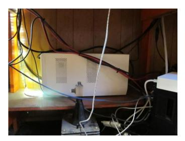
Also on this side of the table is a large truck battery and it is connected to the other side of the 12 volt bus. This allows for continuous 12 volt power for an extended period of time during power failures. The bat-
