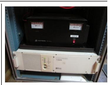
does not supply power for things such as the linear amplifiers. Also one should be careful not to plug in anything like an electric heater to an outlet marked UPS. It uses four 7ah batteries.
