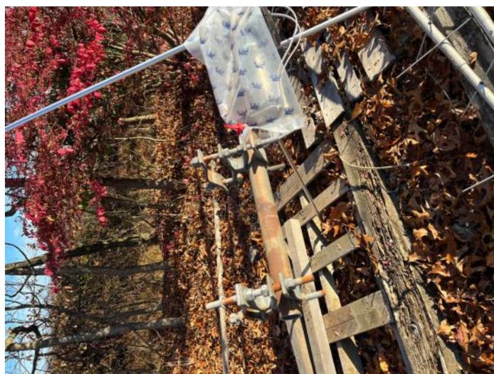
Between the section of iron pipe and the Station Master clamp there was much more weight at the bottom of the antenna than there would be otherwise. This worked as an advantage because when we roped the antenna up the tower, the antenna naturally "Wanted to" keep vertical!
