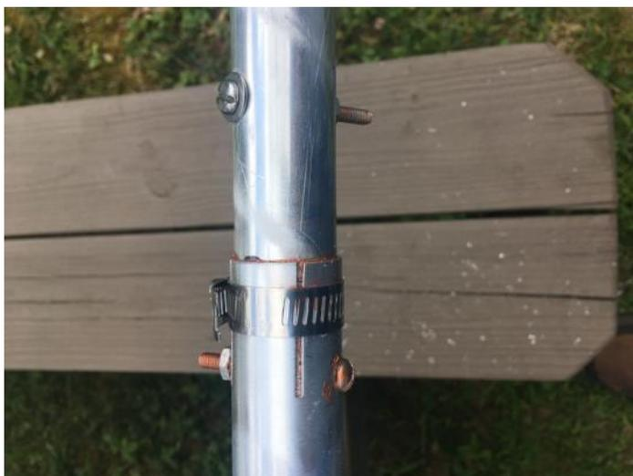
We had a spare "Station Master" antenna clamp to attach the antenna to the tower side arm. The factory mount on the antenna will not accommodate a 2-inch mast, which is what is on the tower side arm. We had some black iron gas pipe at the clubhouse so I cut a section off to use as a go-between, between the antenna mount and the side arm/Station Master clamp.
